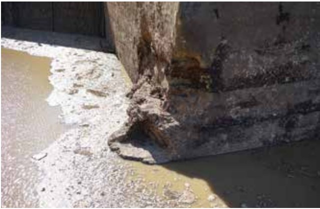
Figure 3.15. UAS documentation of infrastructure conditions at the otherwise inaccessible base of a hydroelectric dam (Maser Consulting)
